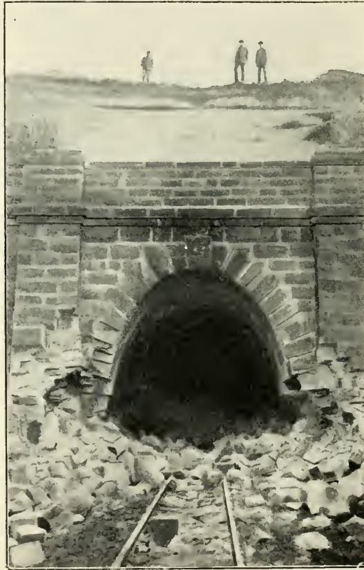
TUNNEL NEAR LAING'S NEK WRECKED BY THE BOERS. South view.
